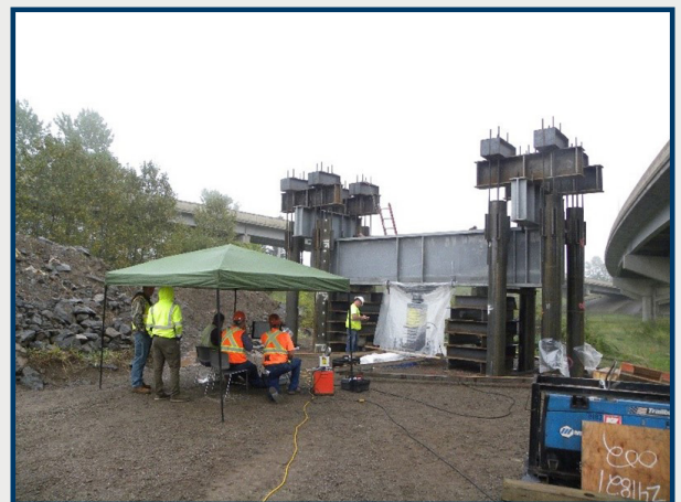
Pile load testing
