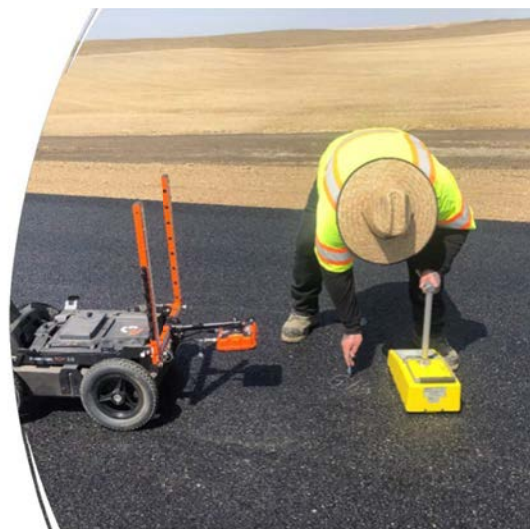
FIGURE 16 What DPS provides for contractor quality control.
