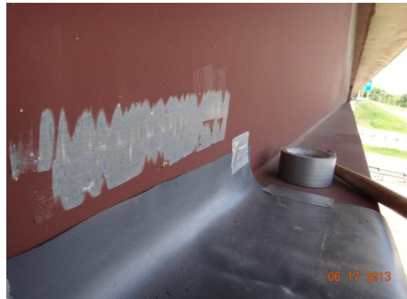
Figure 3.4.62: Bridge #27080 sampling location
