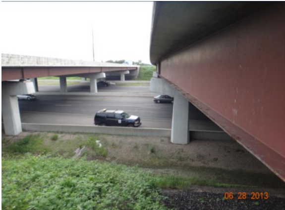
Figure 3.4.44: Bridge #19824 with roadway
