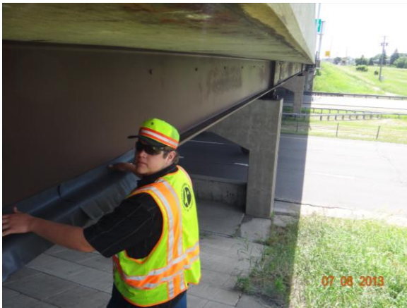
Figure 3.4.38: Bridge #9012 with roadway
