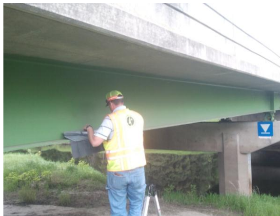
Figure 3.1.14: Bridge #6503 sampling location with waterway
