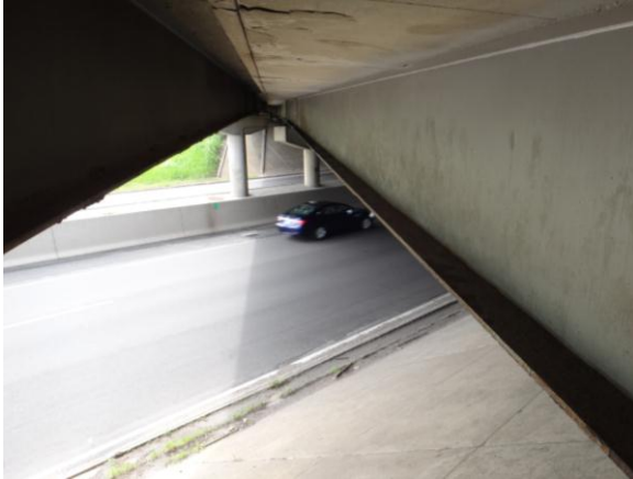
Figure 3.4.9: Bridge #27038 with roadway
