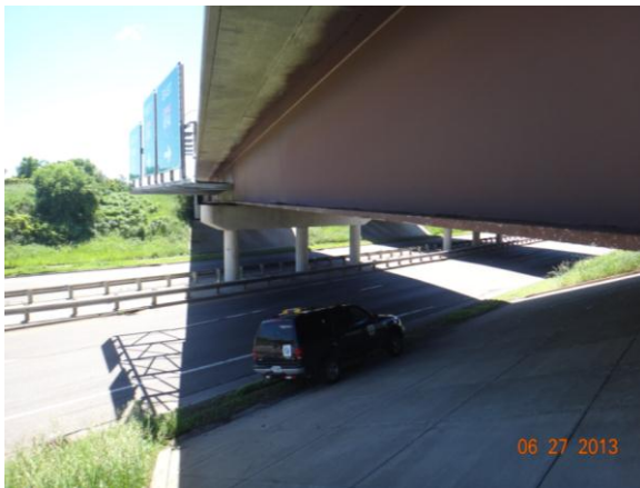
Figure 3.4.49: Bridge #19037 with roadway
