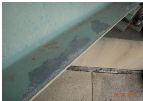
Figure 3.1.6: Bridge #9188 sampling location
