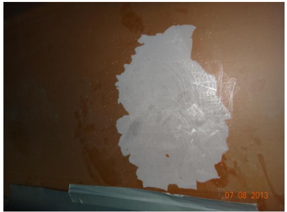
Figure 3.4.35: Bridge #9352 sampling location
