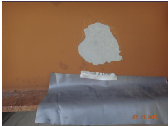
Figure 3.4.12: Bridge #27033 sampling location
