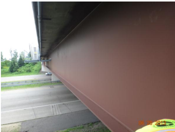
Figure 3.4.24: Bridge #82844 with roadway
