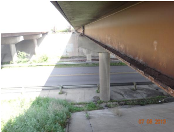
Figure 3.4.34: Bridge #9352 with roadway
