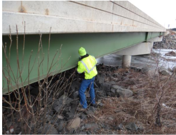
Figure 3.1.11: Bridge #9339 sampling location with waterway
