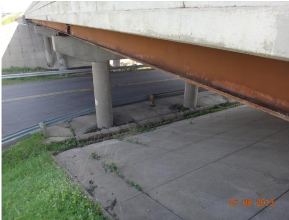
Figure 3.4.32: Bridge #9351 with roadway
