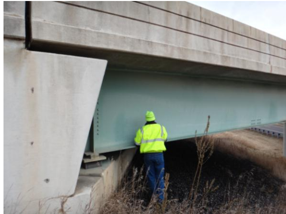
Figure 3.1.4: Bridge #9838 sampling location with roadway
