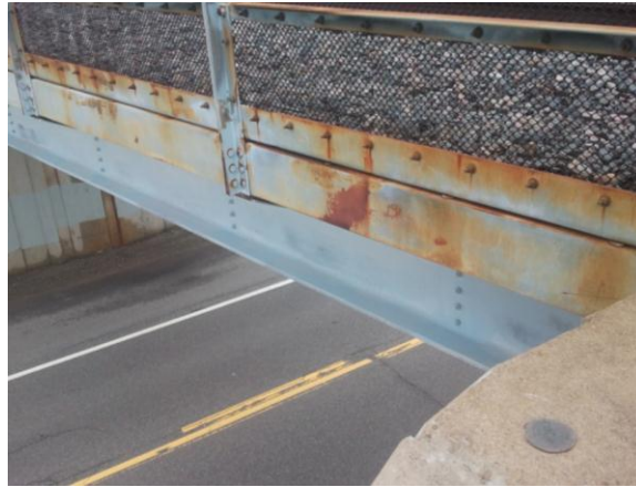
Figure 3.1.13: Bridge #9186 with roadway
