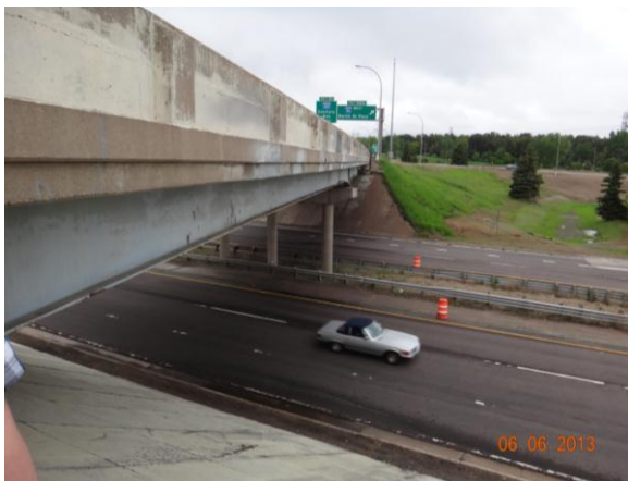
Figure 3.4.28: Bridge #82814 with roadway
