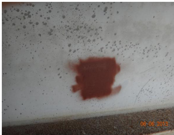
Figure 3.4.29: Bridge #82814 sampling location
