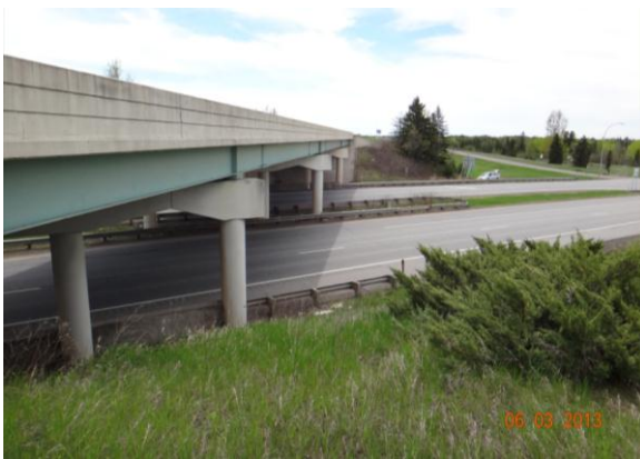
Figure 3.1.5: Bridge #9188 with roadway
