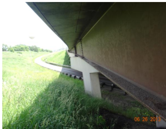
Figure 3.4.57: Bridge #19884 sampling location with roadway
