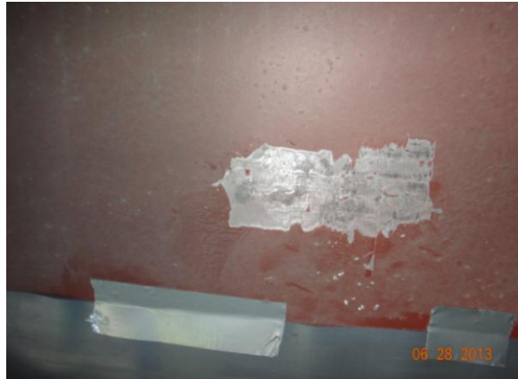
Figure 3.4.45: Bridge #19824 sampling location
