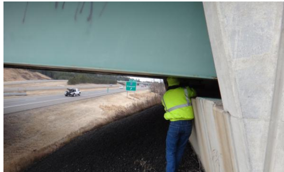
Figure 3.1.3: Bridge #9837 sampling location with roadway
