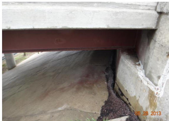
Figure 3.3.4: Bridge #67801 sampling location with roadway shoulder
