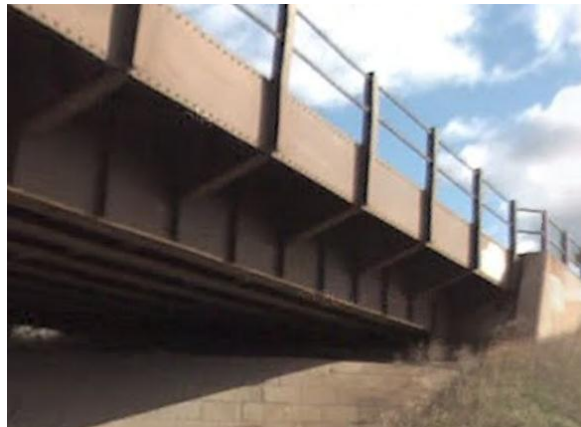
Figure 3.2.2: Bridge #9480 sample location
