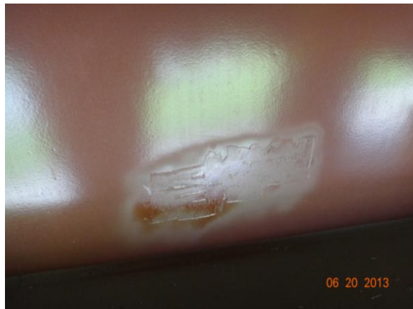
Figure 3.4.20: Bridge #27734 sampling location
