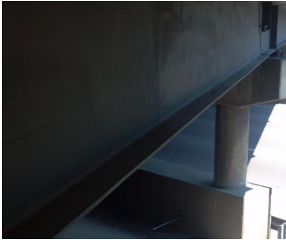
Figure 3.4.1: Bridge #27869 with roadway
