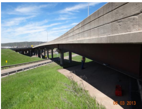
Figure 3.1.7: Bridge #69808A with roadway
