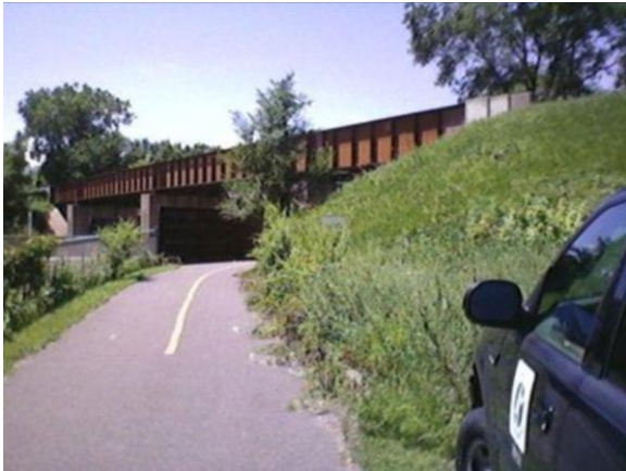
Figure 3.4.36: Bridge #9390 with roadway
