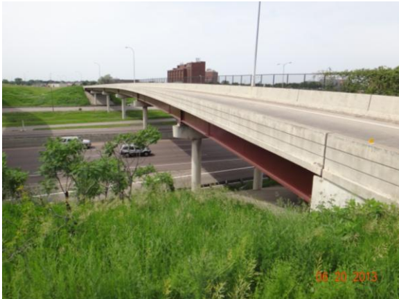
Figure 3.4.17: Bridge #27913 with roadway
