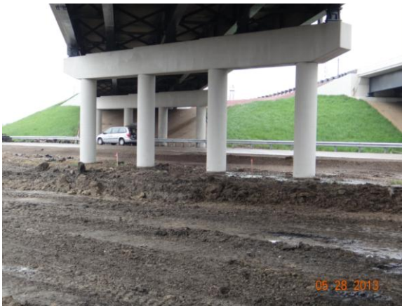
Figure 3.3.2: Bridge #53820 with roadway
