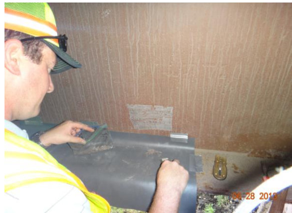
Figure 3.4.43: Bridge #19823 sampling location
