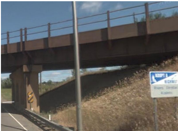
Figure 3.2.1: Bridge #9480 with roadway
