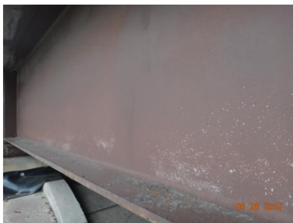
Figure 3.4.31: Bridge #82832 sampling location
