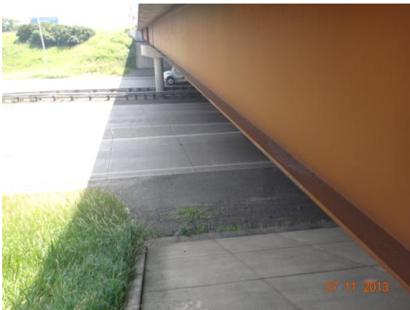
Figure 3.4.11: Bridge #27033 with roadway
