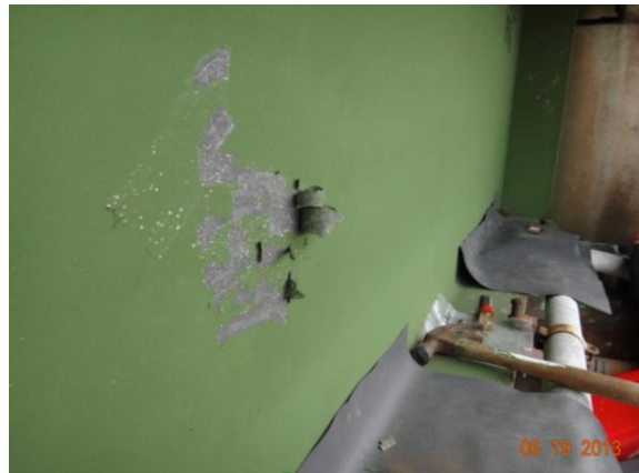
Figure 3.4.59: Bridge #27517 sampling location
