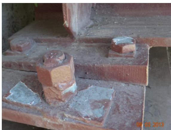
Figure 3.1.10: Bridge #69811 sampling location
