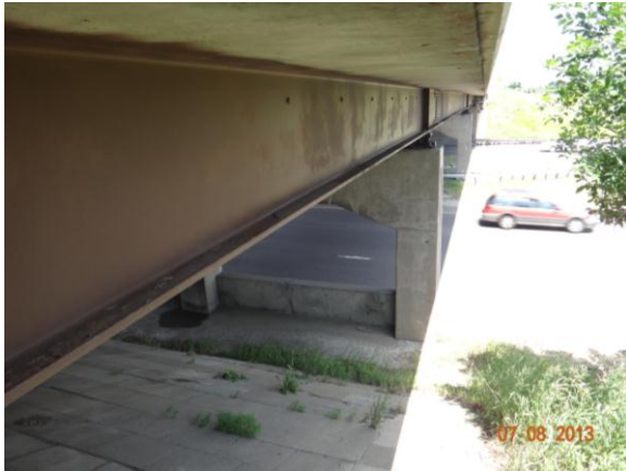
Figure 3.4.40: Bridge #9013 with roadway
