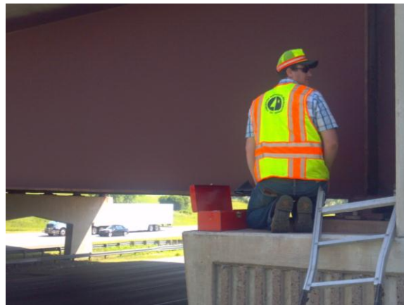
Figure 3.4.22: Bridge #82846 sampling location with roadway
