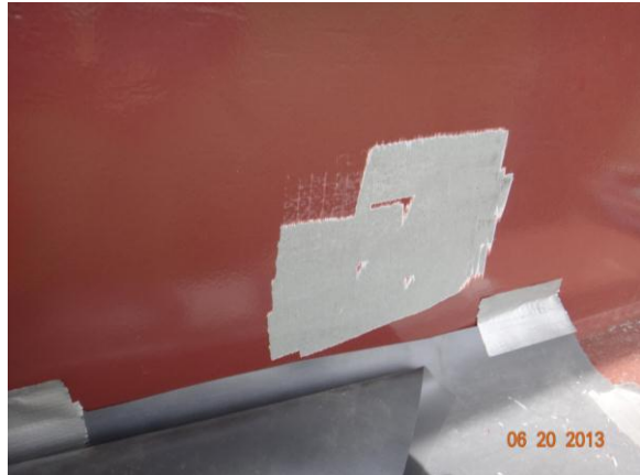
Figure 3.4.18: Bridge #27913 sampling location
