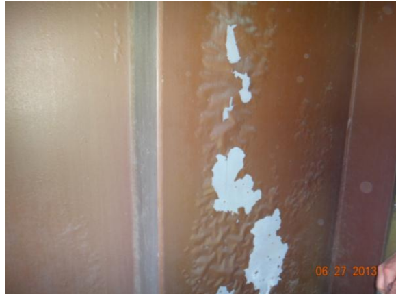
Figure 3.4.52: Bridge #19832 sampling location
