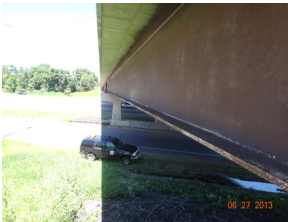
Figure 3.4.53: Bridge #19854 with roadway
