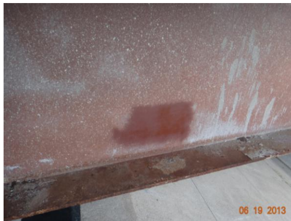
Figure 3.4.64: Bridge #27014 sampling location
