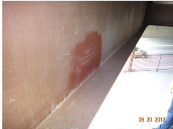
Figure 3.4.21: Bridge #27924 sampling location with roadway
