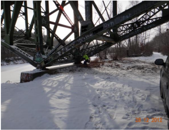
Figure 3.1.1: Bridge #5718 with waterway
