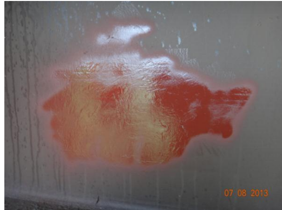
Figure 3.4.41: Bridge #9013 sampling location
