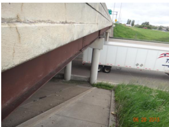
Figure 3.4.30: Bridge #82832 with roadway
