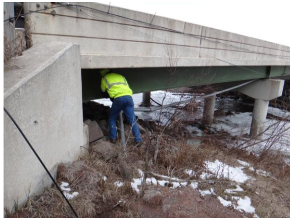
Figure 3.1.12: Bridge #9341 sampling location with waterway
