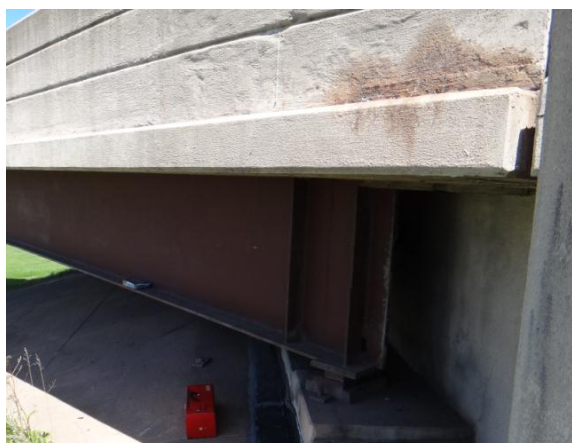
Figure 3.1.8: Bridge #69808A sampling location
