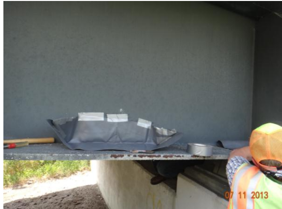
Figure 3.4.6: Bridge #27031A sampling location
