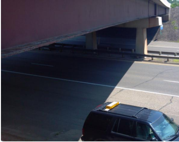
Figure 3.4.13: Bridge #82849 with roadway
