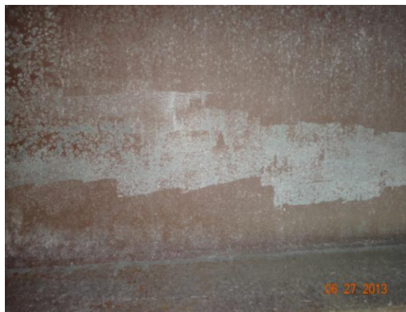
Figure 3.4.54: Bridge #19854 sampling location
