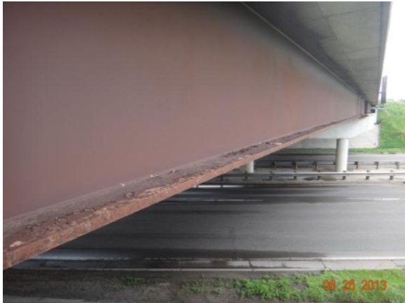
Figure 3.4.55: Bridge #19038 with roadway
