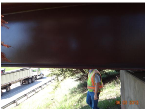
Figure 3.1.9: Bridge #69811 with roadway
