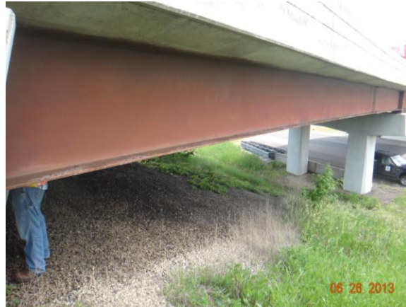
Figure 3.4.48: Bridge #19889 sampling location with roadway
