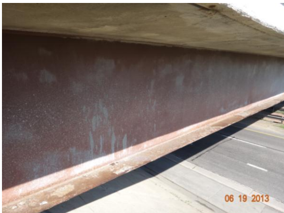
Figure 3.4.63: Bridge #27014 with roadway
