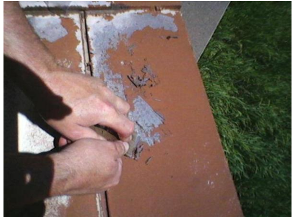
Figure 3.4.37: Bridge #9390 sampling location
