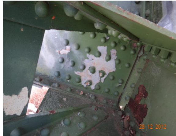
Figure 3.1.2: Bridge #5718 sampling location
