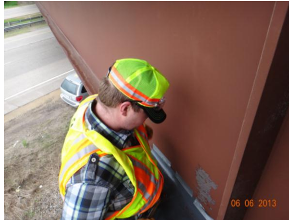
Figure 3.4.26: Bridge #82848 sampling location with roadway
