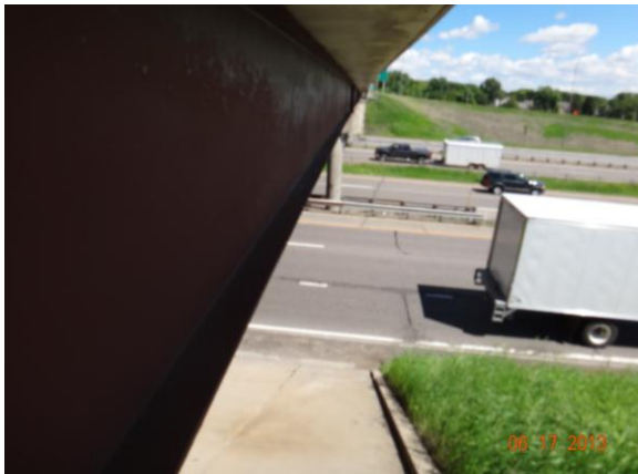
Figure 3.4.61: Bridge #27080 with roadway
