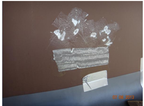
Figure 3.4.39: Bridge #9012 sampling location
