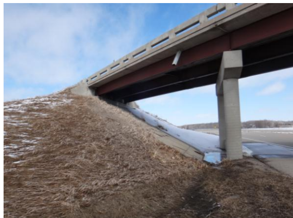
Figure 3.2.3: Bridge #73818 with roadway
