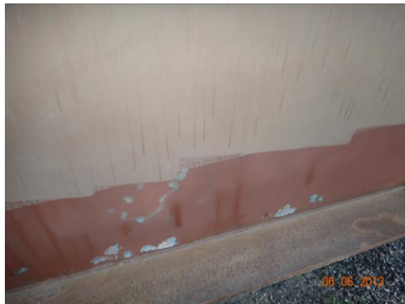
Figure 3.4.47: Bridge #19882 sampling location
