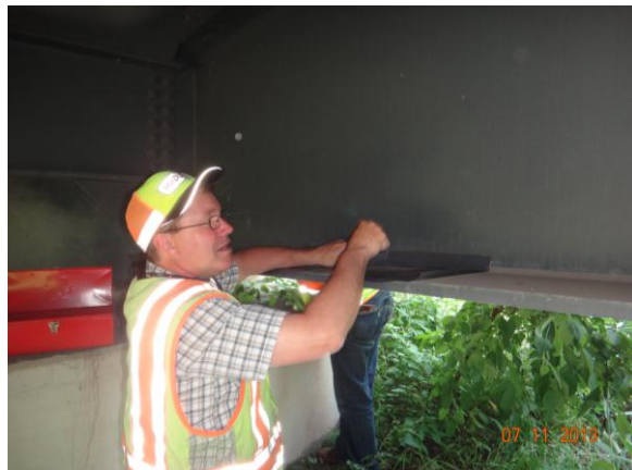
Figure 3.4.8: Bridge #27031B sampling location
