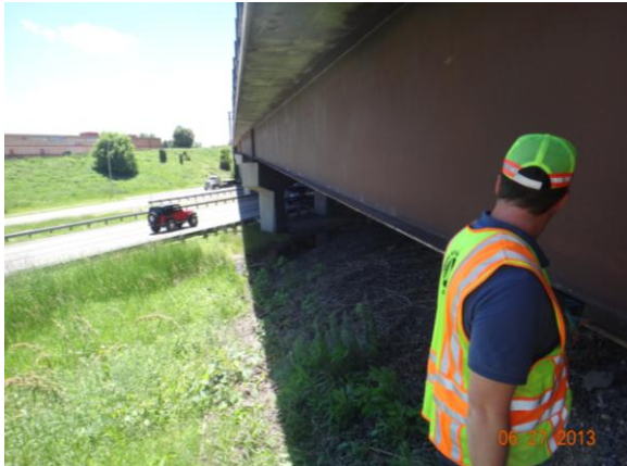
Figure 3.4.51: Bridge #19832 with roadway
