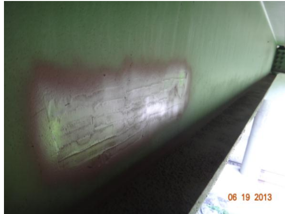
Figure 3.4.58: Bridge #27513 sampling location with roadway
