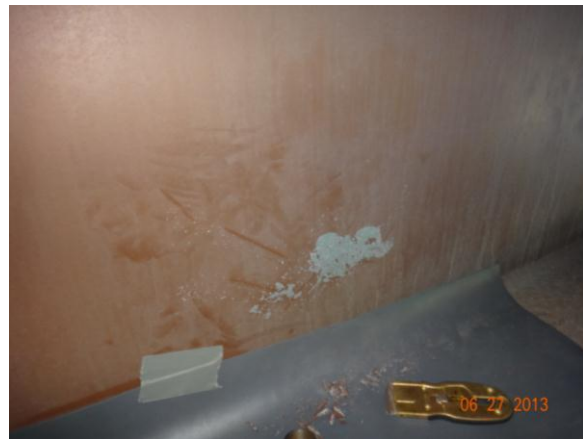
Figure 3.4.50: Bridge #19037 sampling location
