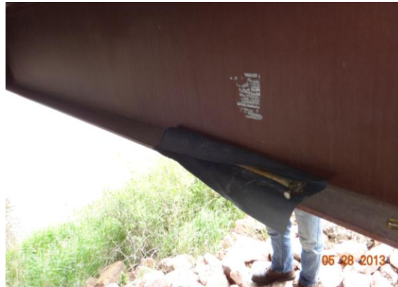
Figure 3.3.1: Bridge #67806 sampling location with waterway
