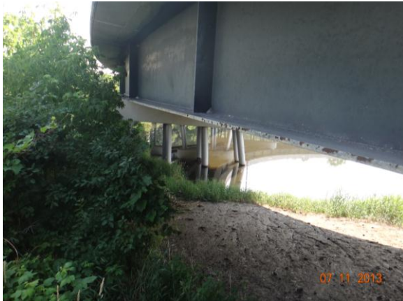
Figure 3.4.5: Bridge #27031A with roadway
