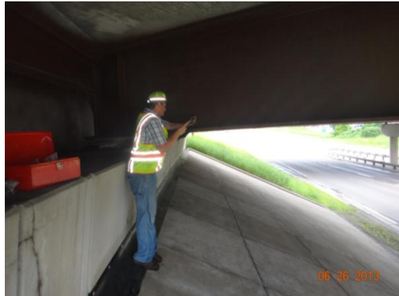
Figure 3.4.56: Bridge #19038 sampling location
