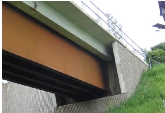
Figure 3.4.23: Bridge #19829 sampling location
