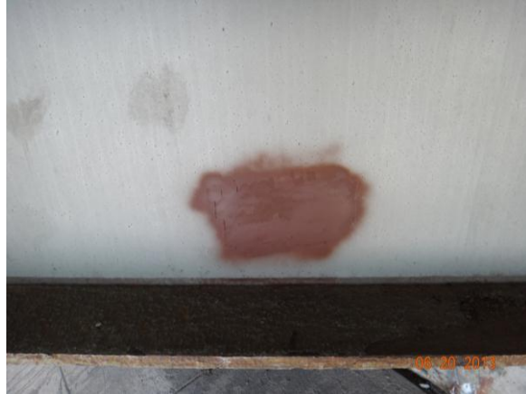
Figure 3.4.10: Bridge #27038 sampling location
