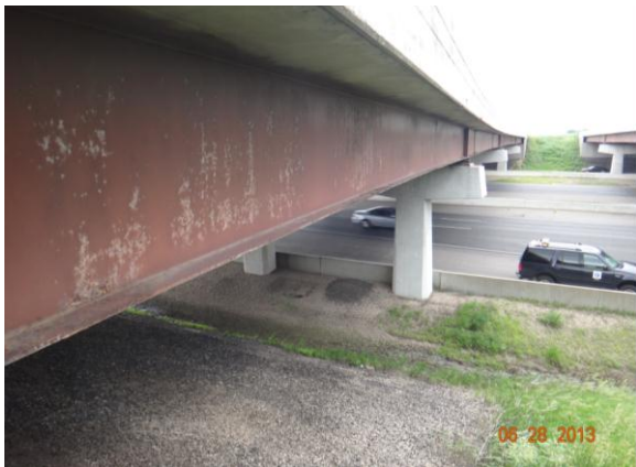
Figure 3.4.42: Bridge #19823 with roadway
