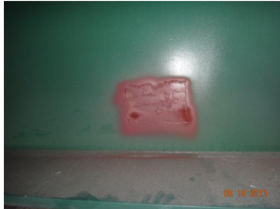
Figure 3.4.60: Bridge #27106 sampling location
