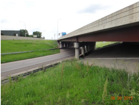
Figure 3.4.19: Bridge #27734 with roadway
