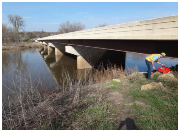
Figure 3.3.5: Bridge #40001 sampling location with waterway
