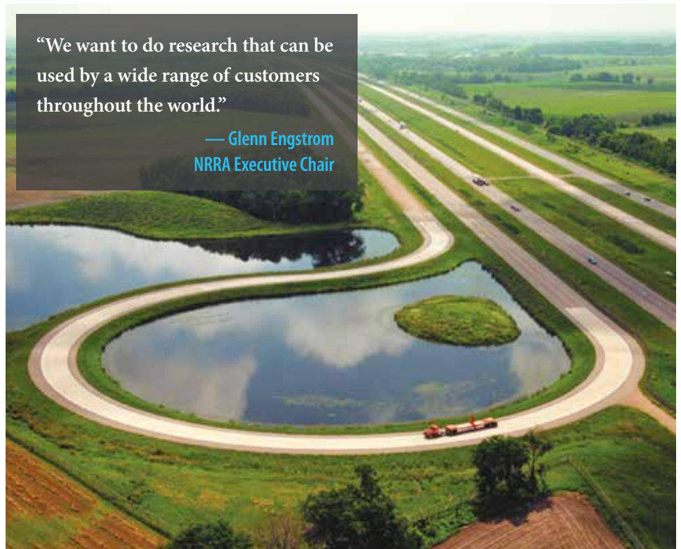
MnROAD's outdoor test tracks include this low-volume, 2.6-mile closed loop that simulates city and county conditions.
