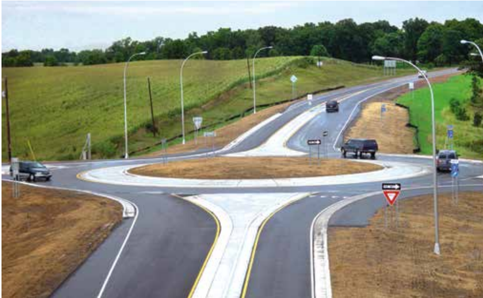
Traffic engineers would like more guidance on how to slow down traffic approaching roundabouts at high speeds. Pictured is a roundabout at Highway 13 and County Road 2 in Scott County before enhancements were made. (Photo courtesy of Scott County)
