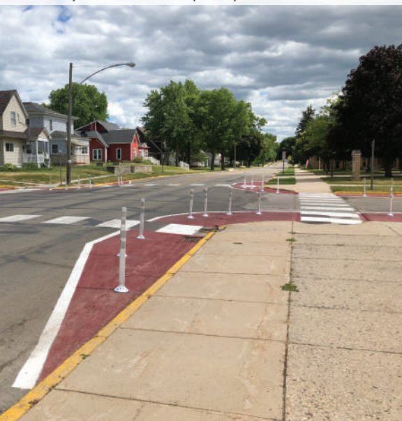
Hwy 22/3rd St temporary curb extension
