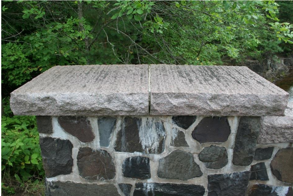
Cap stones on end posts, detail view
