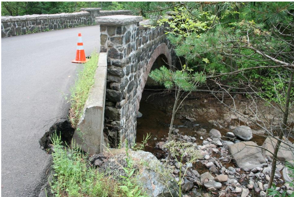
Concrete retaining wall on north side of bridge, view facing south
