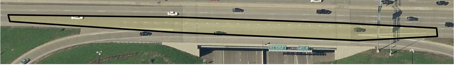
Figure 2: This figure highlights where and what the auxiliary buffer lane is (I-494 and MN 100)
