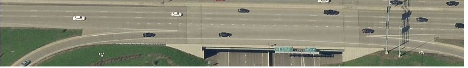
Figure 1: An interchange section that contains an auxiliary buffer lane (I-494 and MN 100)
