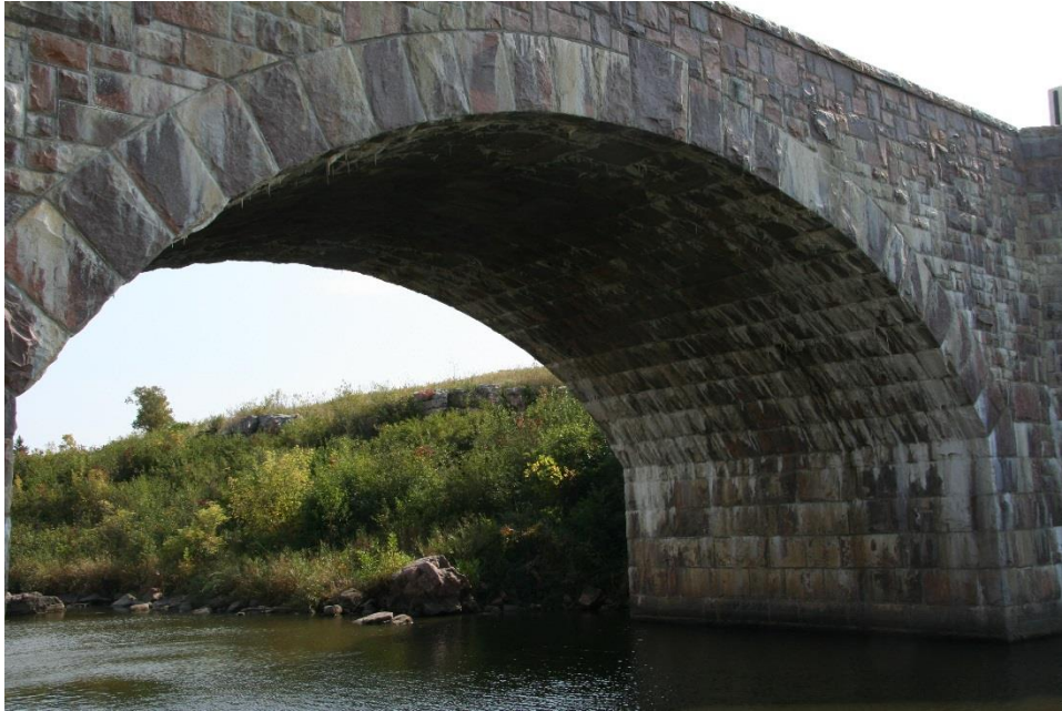
View facing southeast
