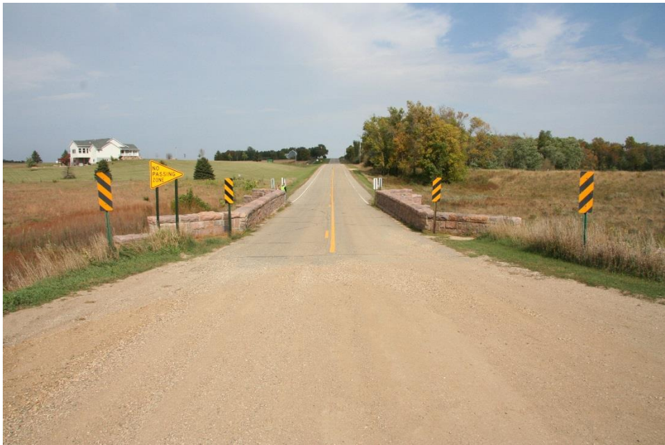
View facing north
