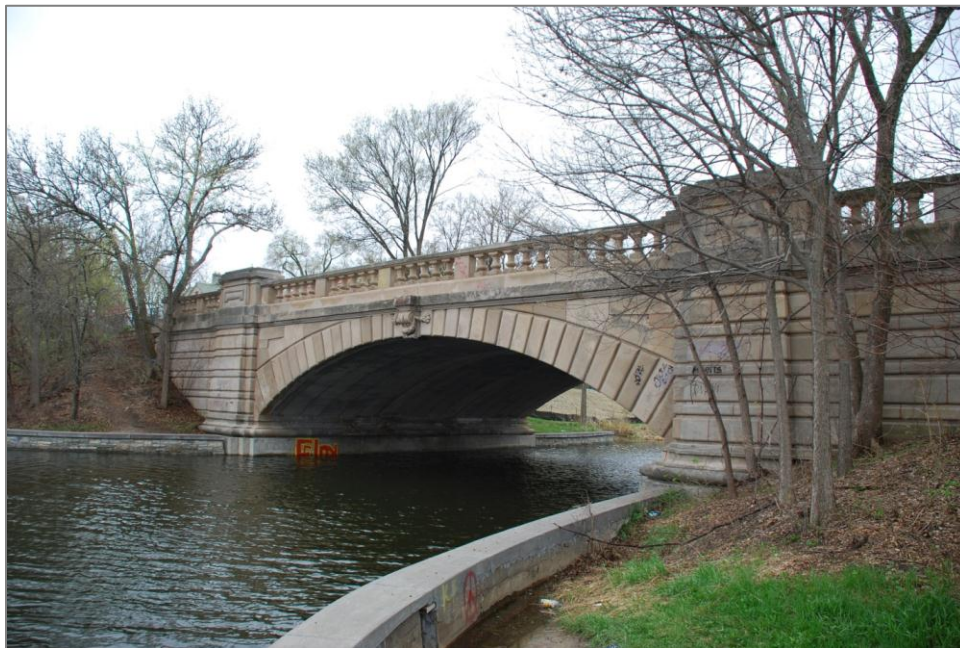
Figure 2. Classical Revival Style Bridge, West Lake of the Isles Parkway over Kenilworth Lagoon, Minneapolis
