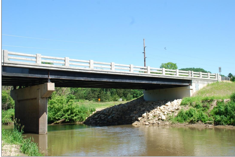
Figure 5. Example of "modern" bridge with unadorned piers and bi-rail railing. Bridge 6679, Sheldon Township, Houston County
