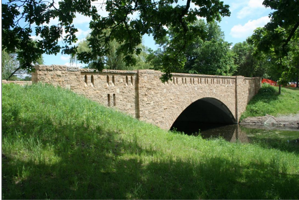
Figure 3. Rustic Style Bridge. Bridge L8560, Phalen Park, St. Paul
