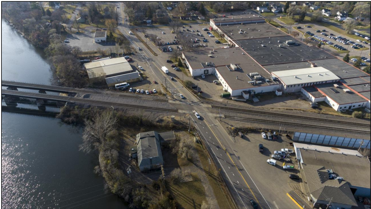
Figure 1. Hwy 47 and BNSF Railway Crossing
