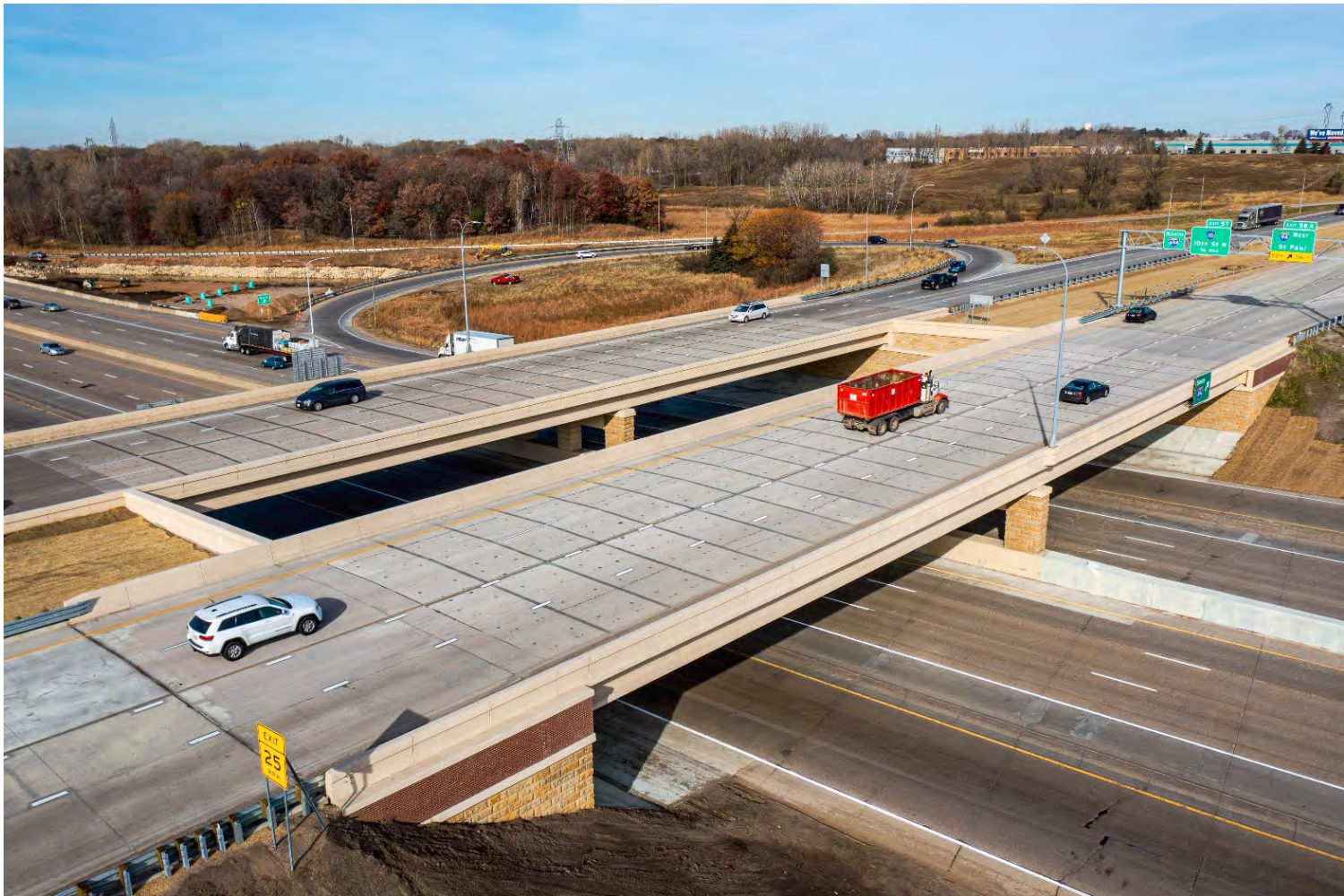
Photo by WSP USA Inc.
