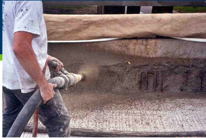
Concrete surface repair
