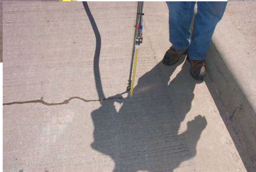
Crack sealing
