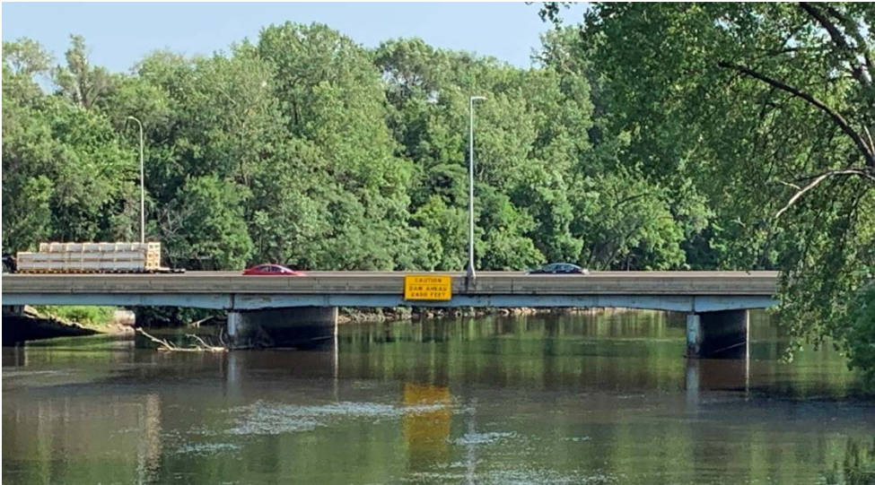
Existing Bridge Site
